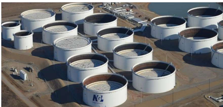
NGL Cushing Crude Oil Storage Tanks
